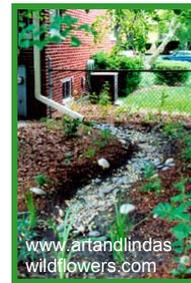
Rain gardens are large basins that collect and hold water that runs off impervious (hard) surfaces like your roof or driveway. The porous nature of the rain garden soil allows the water to infiltrate into the ground. While the plants, mulch and soil, in the garden trap pollutants and sediment.
