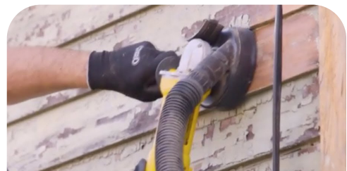
Avoid abrasive and damaging cleaning methods such as orbital sanders. Scrape peeling paint by hand.
