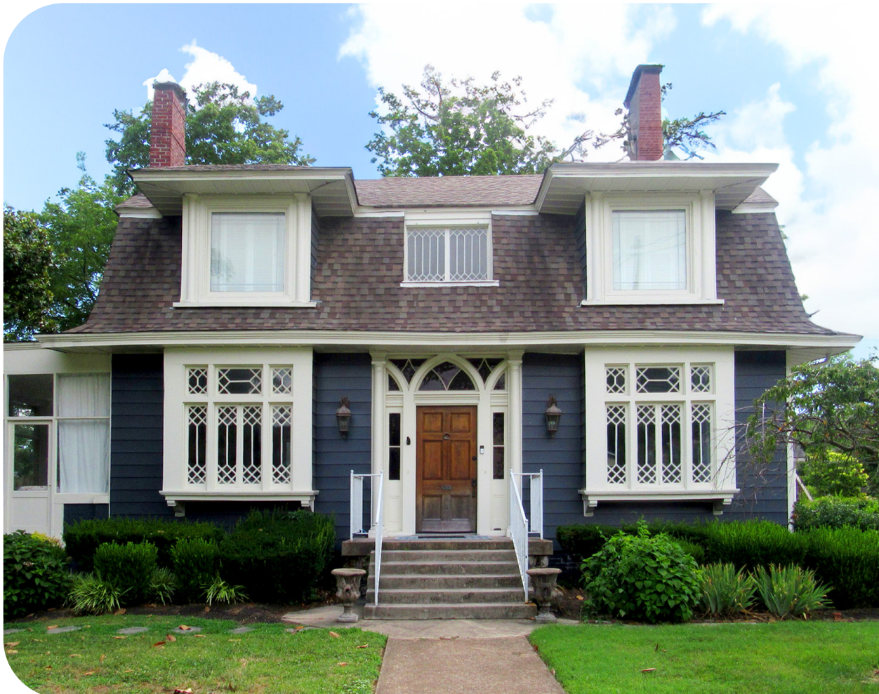
The home at 112 S. Hatton Ave. retains its original mansard roof and features intricate muntins on its window sashes.
