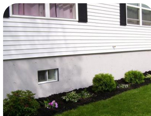
Do not paint masonry foundation surfaces unless historically painted.
