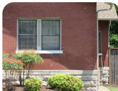
Retain and preserve masonry foundation. (325 W Main St.)
