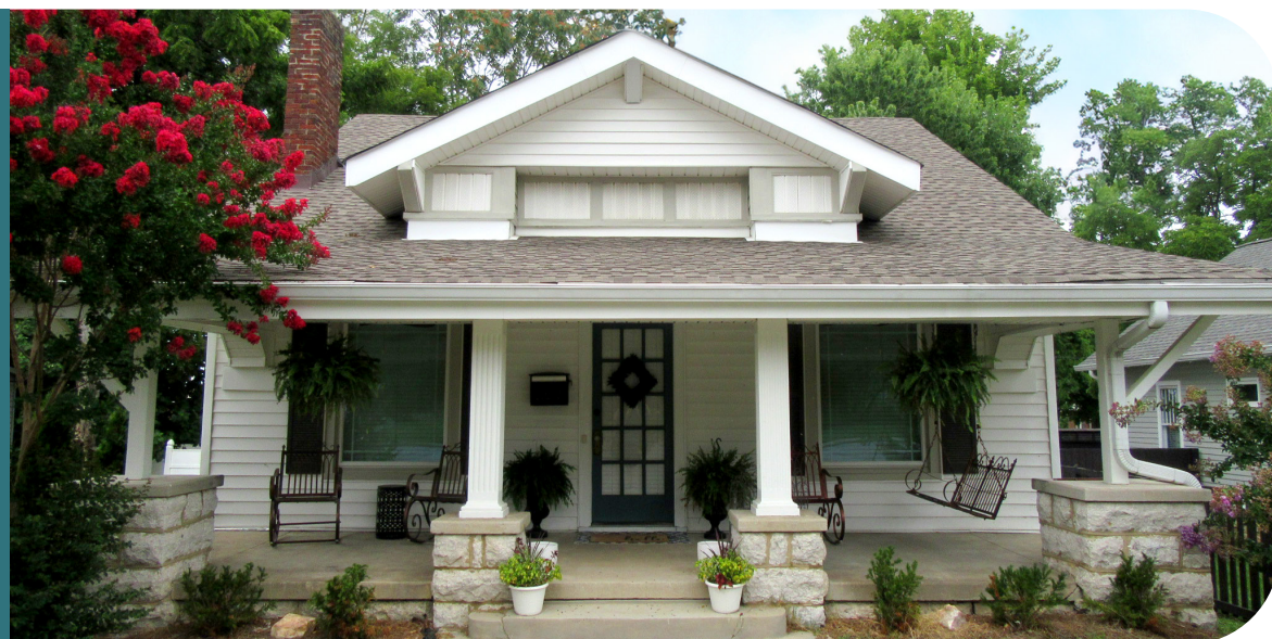
The home at 207 E. Spring St. features a bonnet style roof with a prominent dormer.
