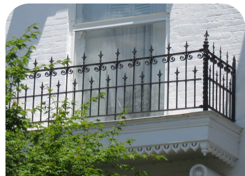
Replace metal with features with identical metal, before substituting. (241 W. Main St.)
