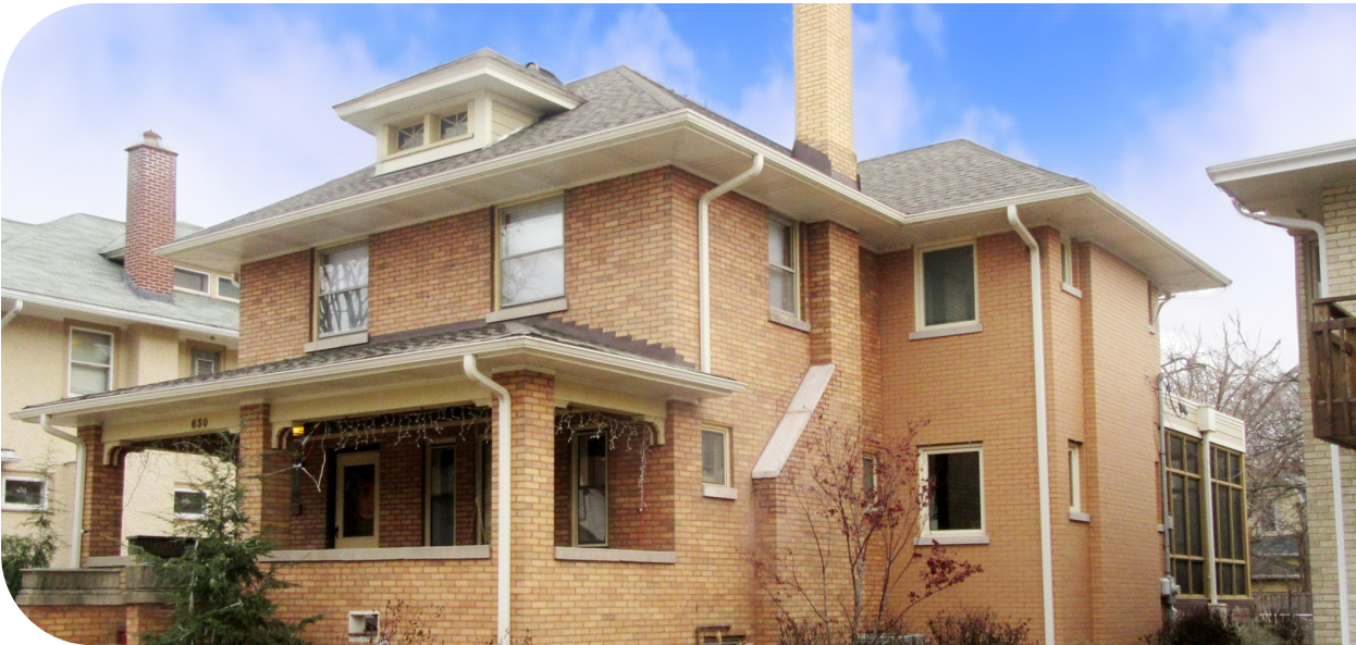
A new addition should be compatible in massing, scale, height, and proportion, as shown on the right.
