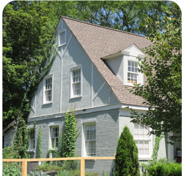
The home at 110 Castle Heights Ave. features a first floor clad in brick, a second floor finish in stucco, and a steeply pitched hipped roof.
